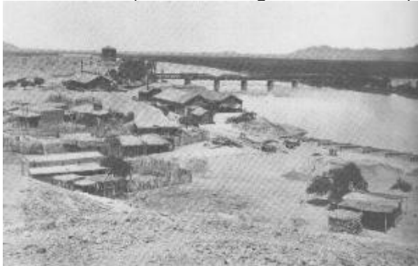
Yuma 1886 (railroad bridge built in 1877)
